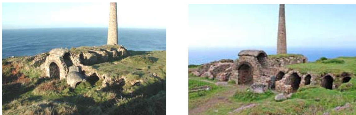
Fig 6: The Botallack labyrinth As works in Cornwall, UK, before (left) and after (right) remediation and site restoration (photo credit: Cornwall County Council).
